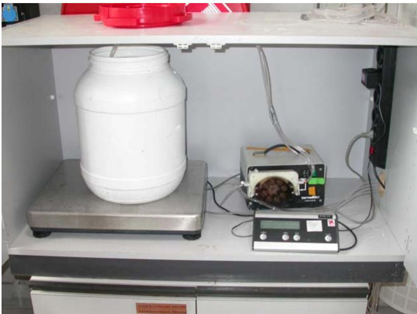
**Figure 8 Box for sheltering of the dosing equipment at a dosing station**
