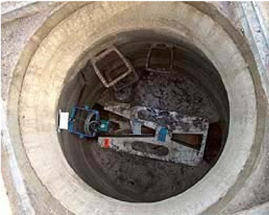
**Figure 13:** *Detailed photo of Parschalls flume with water level meter installed in manhole*
