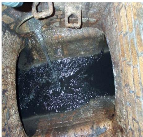
**Figure 2:** *House connection connected to manhole*
