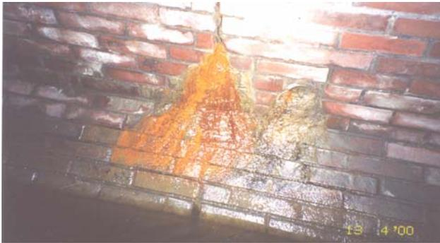
Figure 3-2: Infiltrated groundwater in an old sewer pipe
